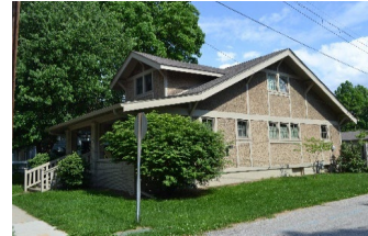
Address 295 W. Rating C Year c. 1925 Style Craftsman Bungalow Notes Good retainage of historic features
