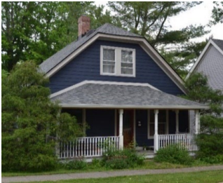
Address 245 N. Rating C Year c. 1900 Style Carpenter-Builder Notes Introduction of new materials, retains basic shape
