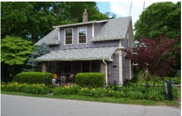
Address 5 N. Rating N Year c. 1870/1910 Style Greek Revival/Craftsman Notes Minor introduction of new materials, features from 1910
