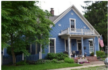
Address 80 N. Rating N Year 1868 Style Carpenter-Builder/Central Gable Notes Minor introduction of new materials
