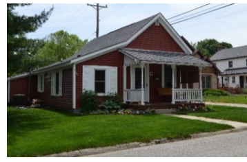
Address 545 W. Rating C Year c. 1900 Style Carpenter-Builder/Gable-front Notes Introduction of new materials, retains basic shape
