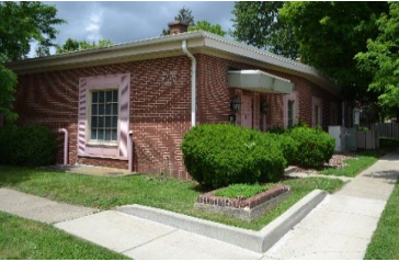
Address 190 S. Rating NC-M Year c. 1960 Style Commercial Building Notes Minor introduction of new materials, retains basic shape
