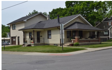
Address 115 W. Rating C Year c. 1925 Style Bungalow Notes Front with good integrity large rear addition, introduction of new materials
