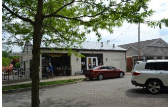
Address 95 E. Rating NC-M Year c. 1965 Style Commercial Building Notes
