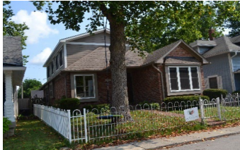
Address 950 W. Rating NC-P Year c. 1920 Style House Notes Significantly altered
