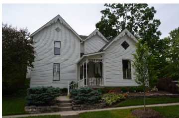
Address 90 N. Rating C Year c. 1885 Style Carpenter-Builder Notes Extensive side addition, new materials
