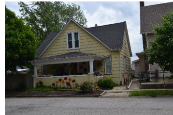
Address 35 E. Rating C Year c. 1870/1910 Style Carpenter-Builder/Central-gable Notes Introduction of new materials, basic shape retained
