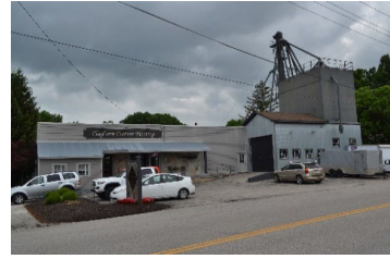
Address 100 N. Rating C Year 1947 Style Grain Elevator/Parapet-front Notes Introduction of new materials, retains basic shape
