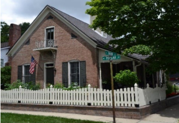
Address 110 N. Rating O Year c. 1880 Style Italianate/Gable-front Notes Minor introduction of new materials, rear addition
