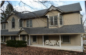
Address 315 N. Rating NC-M Year 1960 Style Notes Extensive remodeling
