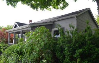
Address 70 E. Rating C Year c. 1940 Style Side-gabled Notes Introduction of new materials, addition/retains basic shape DEMOLISHED 2022
