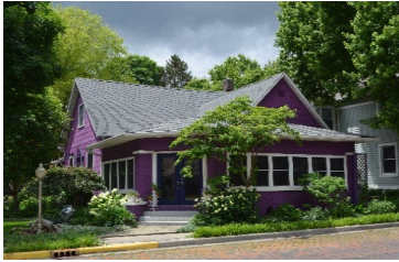
Address 210 N. Rating C Year c. 1890/1915 Style Gabled-ell/Carpenter-Builder Notes Introduction of new materials, retains basic shape
