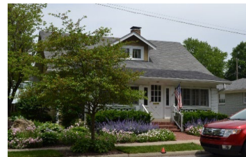
Address 290 W. Rating C Year c. 1920 Style Bungalow Notes Introduction of new materials, porch enclosure
