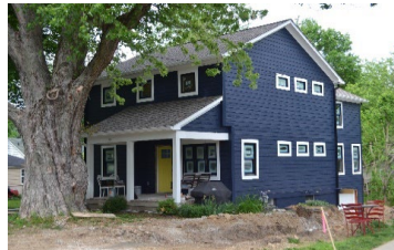
Address 335 S. Rating NC-P Year 1942/2021 Style Notes Substantial remodeling
