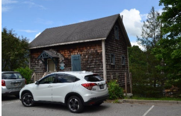
Address N/A Rating NC-M Year c. 1980 Style Commercial Notes DEMOLISHED 2021
