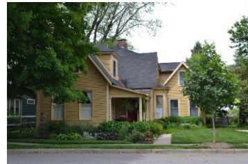
Address 260 W. Rating N Year c. 1885 Style Carpenter-Builder Notes Minor introduction of new materials/additions
