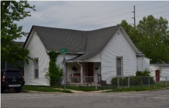
Address 190 W. Rating C Year c. 1890 Style T-plan Notes Introduction of new materials, addition/retains basic shape
