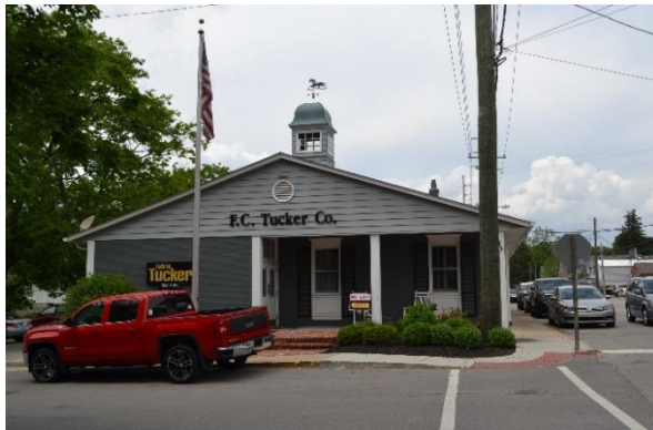
Noteworthy are Zionsville's many late Colonial Revival-styled buildings. While some modifications have been made to the former United States Post Office at 150 W. Cedar, early Colonial architecture was clearly the inspiration for its window surrounds and fluted porch columns. The Colonial Revival lantern capping the roof is topped by a copper roof and weathervane.
